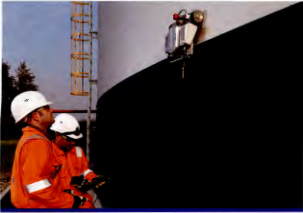
Figure 2. Radio controlled, waterproof, and free climbing, Rosen's tank inspection crawler performs a wide range of tank wall inspections.
