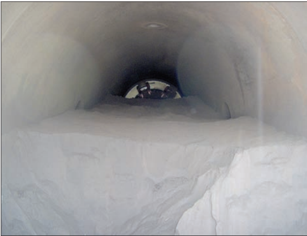
Fig. 3. Receiver filled with black powder.
