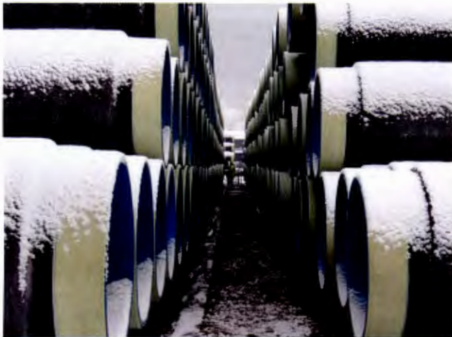
Figure 7. Capped pipes in storage yard.
