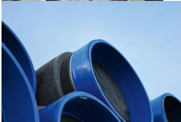
Figure 13 and 14: Capped pipes in storage yards
