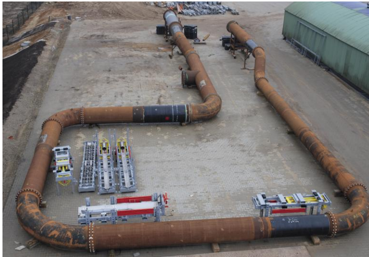
Figure 7: Pump test loop for 32"/42" multi-diameter tools
