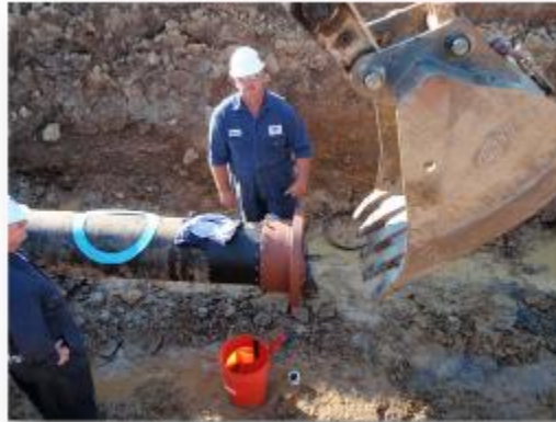
Install flanges for pack-off assembly and insertion of cleaning/tow pig.
