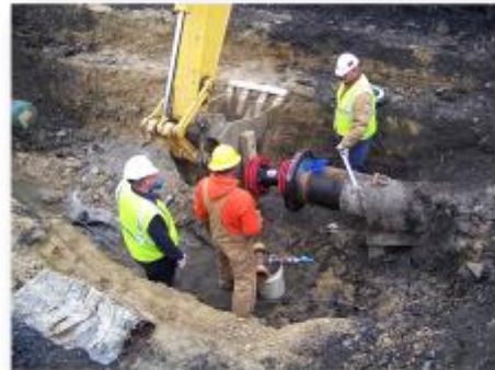
Install flanges for pack-off assembly and insertion of cleaning/tow pig.
