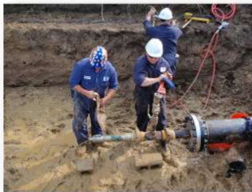
Assemble Pack-off for Propelling Toe Pig to Opposite Ends
