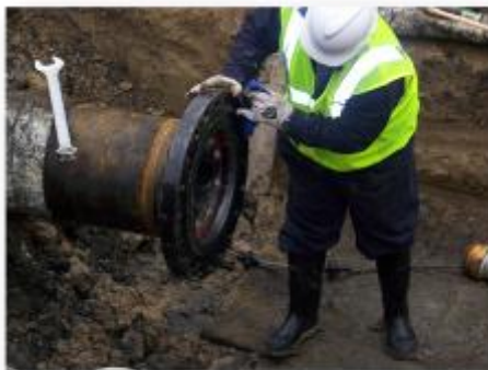
Install flanges for pack-off assembly and insertion of cleaning/tow pig.
