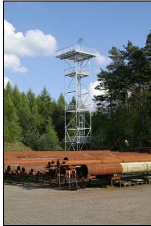
Figure 8: RSS test facility at ROSEN Technology and Research Centre (RTRC), Germany.
